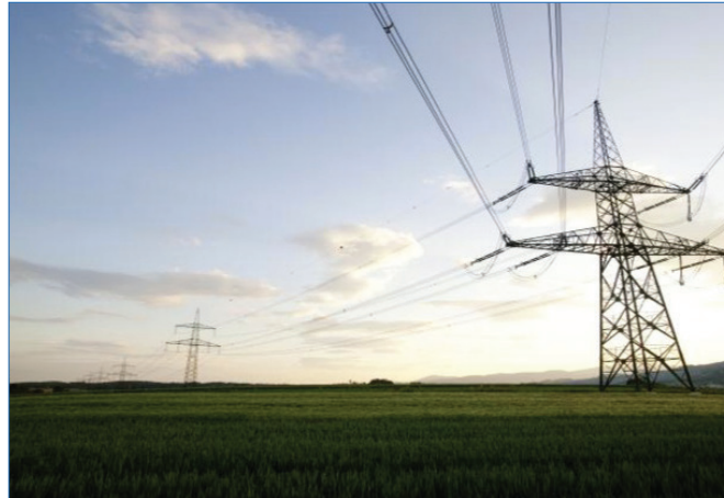
400kV corner mast with OPGW earthwire
